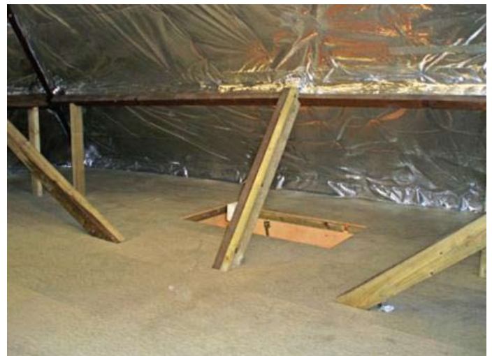
The finished loft
